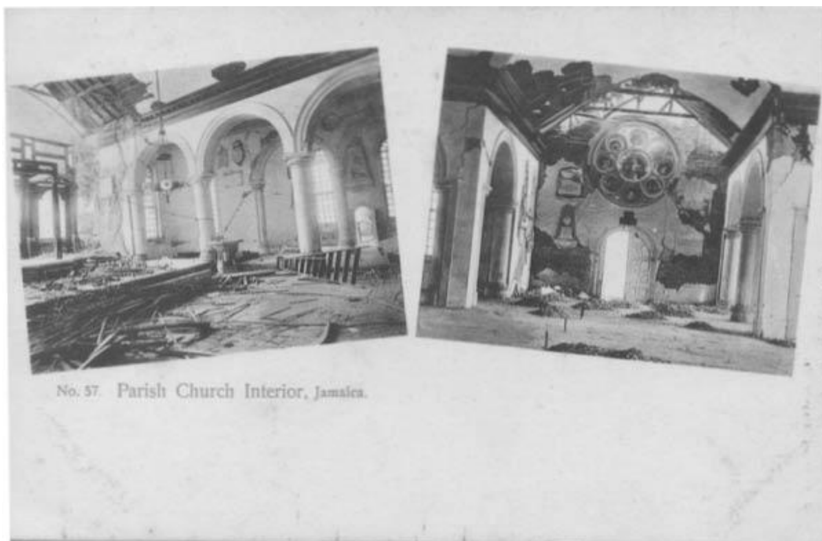
Cleary – Kingston Parish Church Interior
